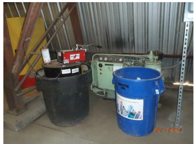
Picture 29 – Warehouse Aerosol Puncture System SAA
