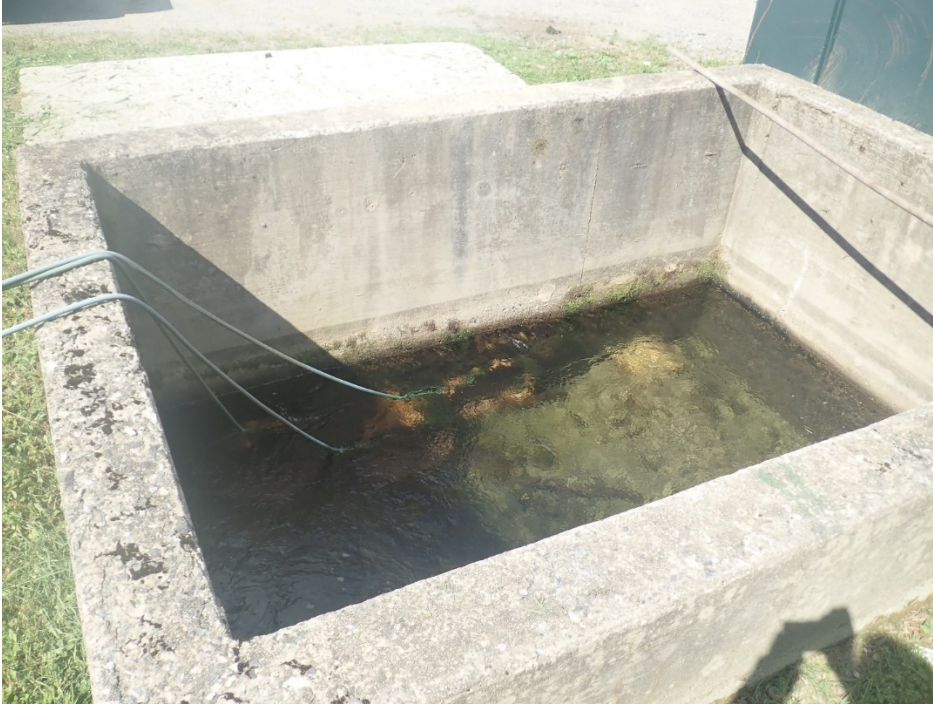
Photo 3. Splitter box distributing water incoming from inlet to three parallel raceway systems. Grey lines are liquid oxygen supplied from a nearby tank.
