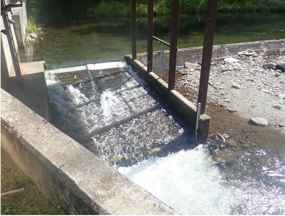
Photo 1. Inlet structure. Water passes through a grate into the system. A rough flow measurement staff is visible at the end of the inlet. Wear is visible on the retaining wall structure. Heavy sedimentation near the wall is the result of high flow conditions.
