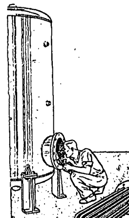
VERTICAL storage heaters work best where the floor space is tight, the head room plentiful. Tube bundle is very short and permits easy handling and maintenance.
