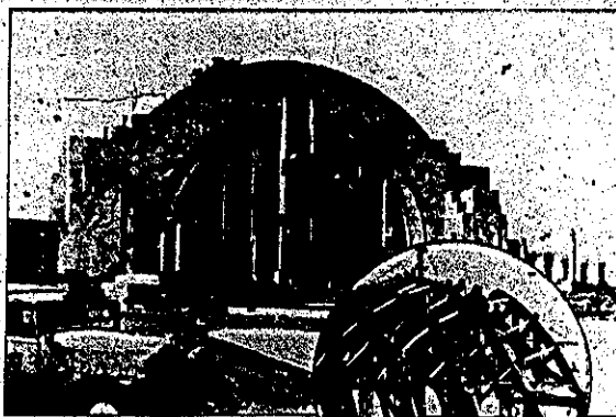
Cincinnati's New Union Terminal Has Thousands of Tons of Steel Structure Rustproofed with Sublimed Blue Lead
