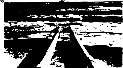
Bechtel Somastic Division have just completed somastic coating a pipe line for the Tide Water Associated Oil Company at Gaviota Canyon. The photograph on the left shows the tracks and the somastic coated pipe before it was launched. The photograph on the right shows a barge in the distance pulling the pipe out from the shore.
