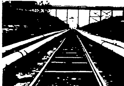
Bechtel Somastic Division have just completed somastic coating a pipe line for the Tide Water Associated Oil Company at Gaviota Canyon. The photograph on the left shows the tracks and the somastic coated pipe before it was launched. The photograph on the right shows a barge in the distance pulling the pipe out from the shore.
