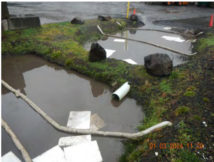
Photo #:47 (DSCN3496) Description: Facing north, photo of Pond 3.
