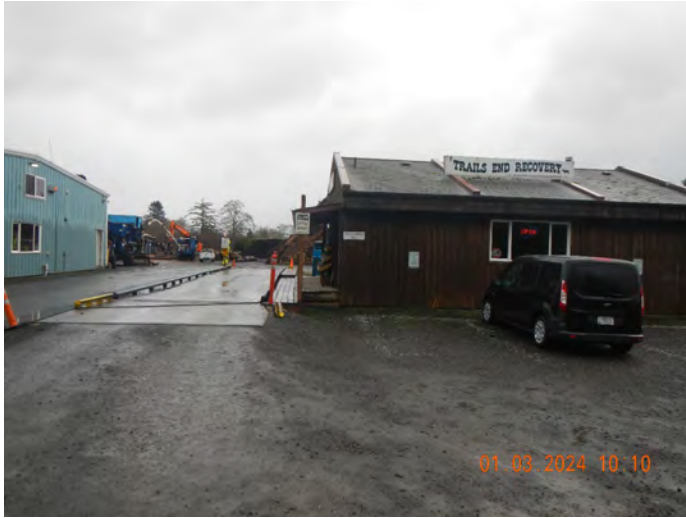
Photo #:01 (DSCN3450) Description: Facing east, photo of the main office building and truck scale/entry.
