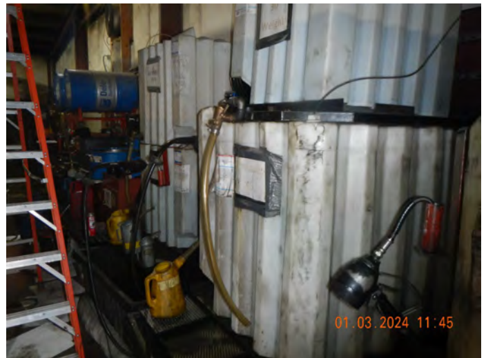
Photo #:56 (DSCN3505) Description: Photo from inside the maintenance shop, oil/lubricant storage area.
