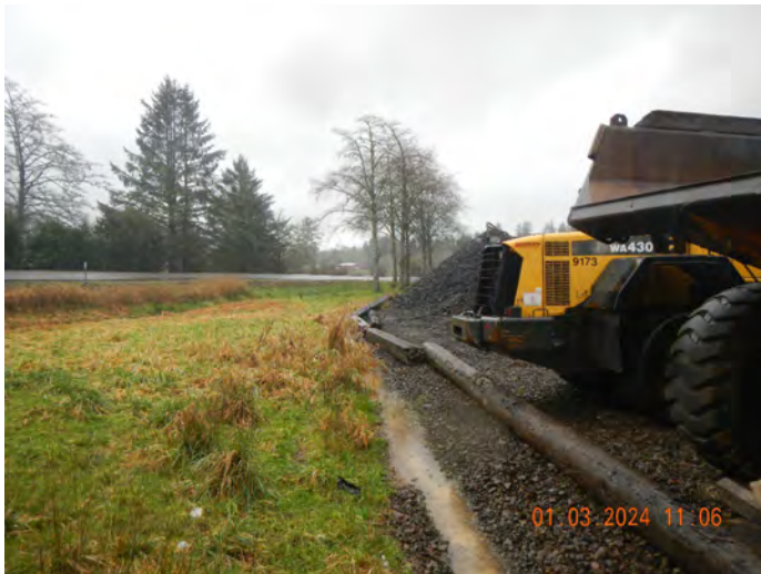
Photo #:27 (DSCN3476) Description: Facing west, photo of southern boundary between the Facility's industrial activities and Highway 101 Alternate.
