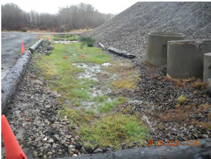
Photo #:19 (DSCN3468) Description: Facing north, photo of Pond 4.
