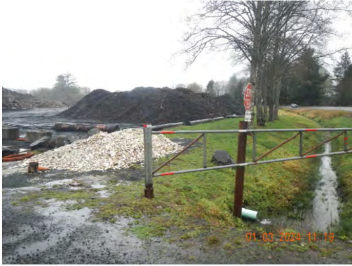
Photo #:37 (DSCN3486) Description: Facing east, photo of the Pond 2 discharge to the unnamed slough.
