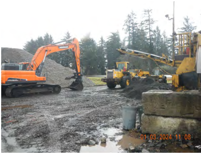
Photo #:29 (DSCN3478) Description: Facing south, photo of a processing/screening area. East of Pond 2.
