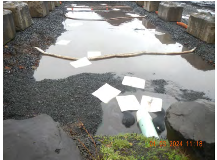
Photo #:36 (DSCN3485) Description: Facing north, photo of Pond 2.
