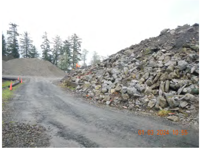
Photo #:18 (DSCN3467) Description: Facing south, photo of the eastern portion of the inerts pile, west of Pond 4.
