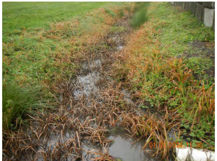
Photo #:48 (DSCN3497) Description: Facing west, photo of upstream location of the Pond 3 outfall, within the roadside drainage ditch.
