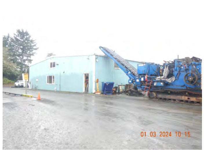
Photo #:02 (DSCN3451) Description: Facing northwest, photo of the maintenance building (shared with Dean Larson Excavation). Woodchipper was staged outdoors awaiting engine replacement.
