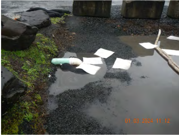
Photo #:33 (DSCN3482) Description: Facing west, photo of Pond 2 outlet cell,
