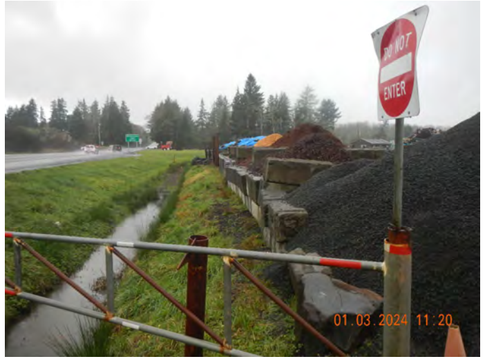
Photo #:38 (DSCN3487) Description: Facing west, photo of the of unnamed ditch upstream of the Pond 2 discharge location.
