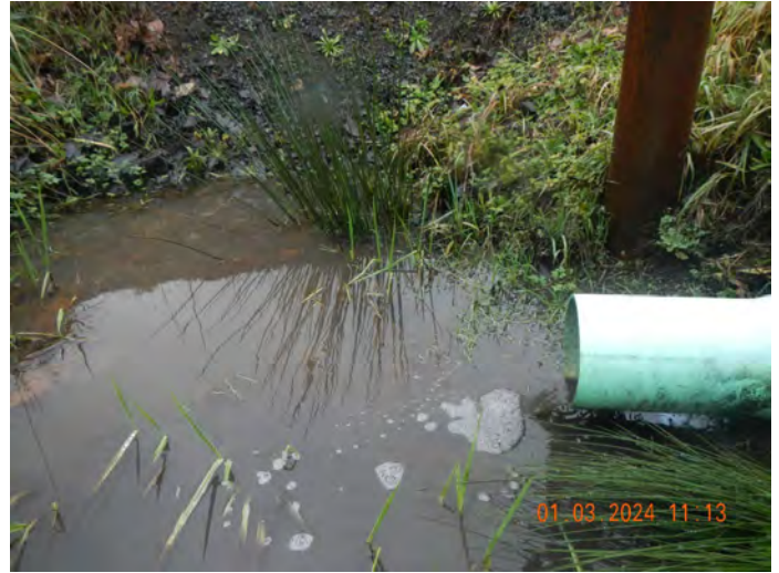
Photo #:34 (DSCN3483) Description: Facing west, photo of Pond 2 discharge. No sheen observed, discharge appeared turbid at the time of inspection.
