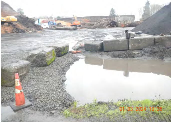
Photo #:09 (DSCN3458) Description: Facing west, photo of the western inlet to Pond 1.
