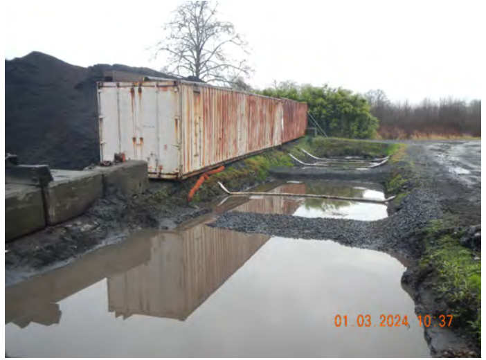
Photo #:10 (DSCN3459) Description: Facing north, photo of the Pond 1 cells/chambers.
