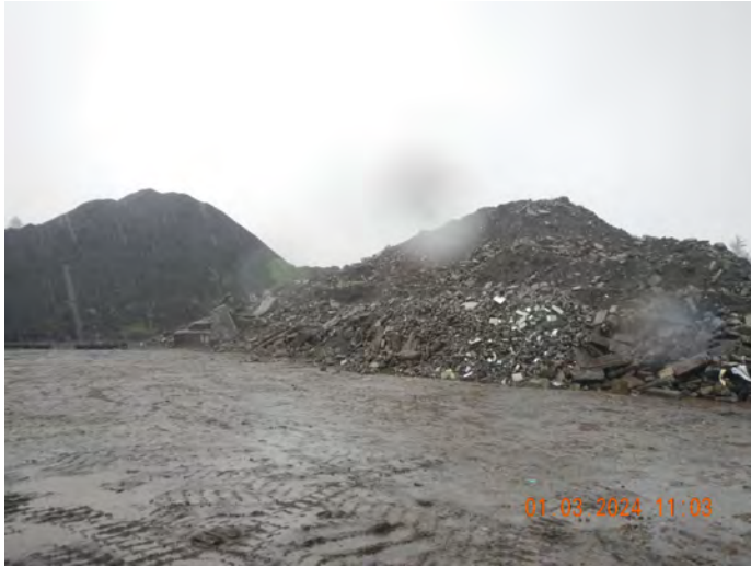
Photo #:25 (DSCN3474) Description: Facing southwest, material stockpile area east of Pond 2.
