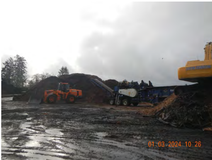
Photo #:07 (DSCN3456) Description: Facing south, photo of the hog fuel processing area.
