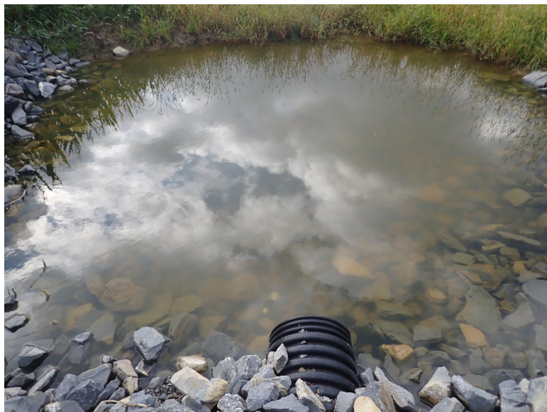
Photograph II.D. Culvert leading to swale at northwest corner of Wetland 19.
