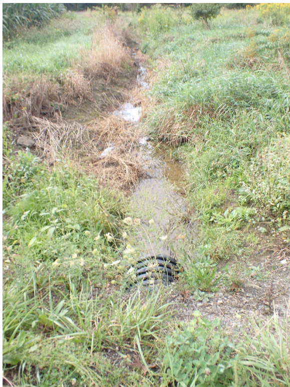
Photograph IV.C. Excavated Wetland 16 tributary. Facing south from Mill Road.
