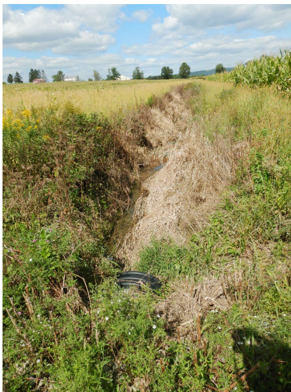
Photograph XVII.D. North extension of UNT-1. Observed while standing on an unnamed path atop a culvert along UNT-1.
