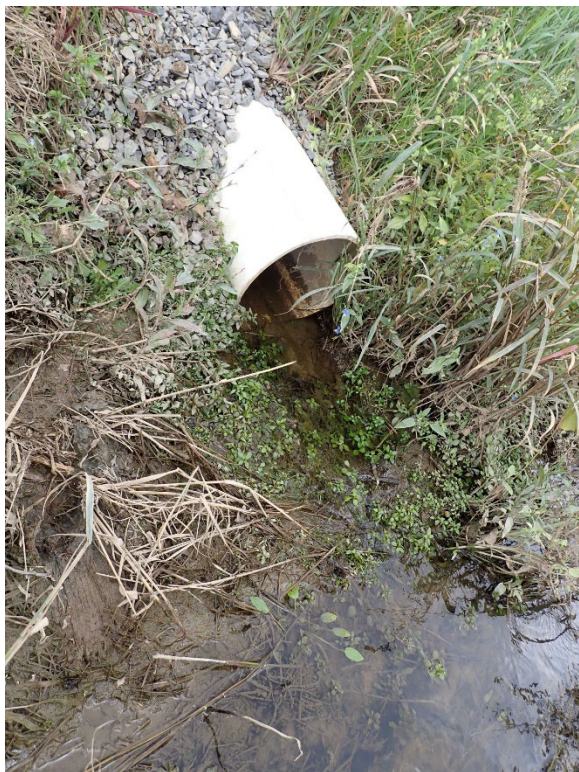
Photograph XI.B. Culvert draining Wetland 8 into Railroad tributary.
