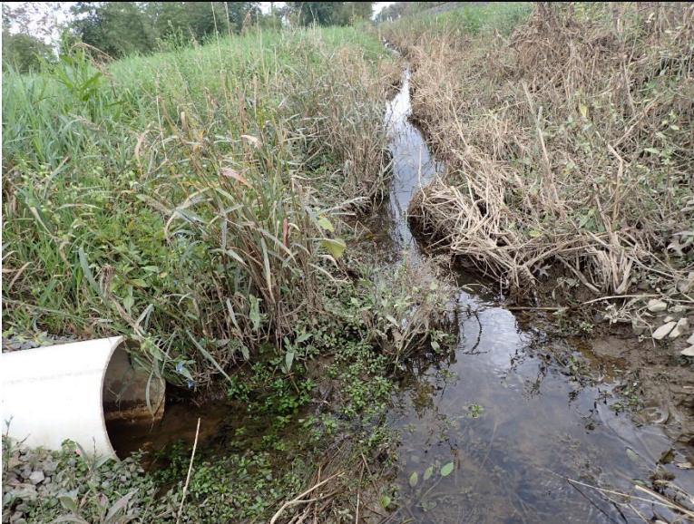
Photograph XI.A. Culvert draining Wetland 8 into Railroad tributary. Facing southeast along Railroad tributary.
