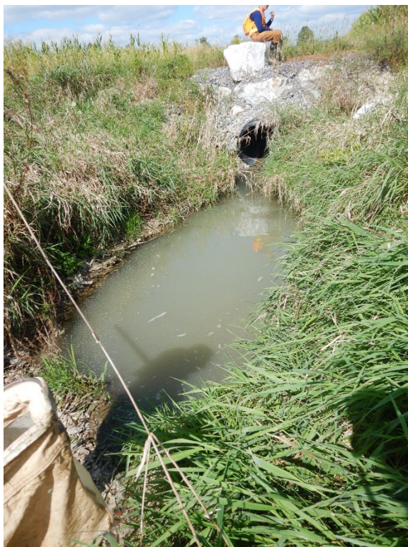
Photograph XVII.B. Swale and culvert along UNT-1. Facing north.
