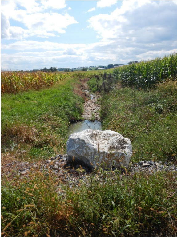
Photograph XVII.E. South extension of UNT-1. Observed while standing on an unnamed path atop a culvert along UNT-1.
