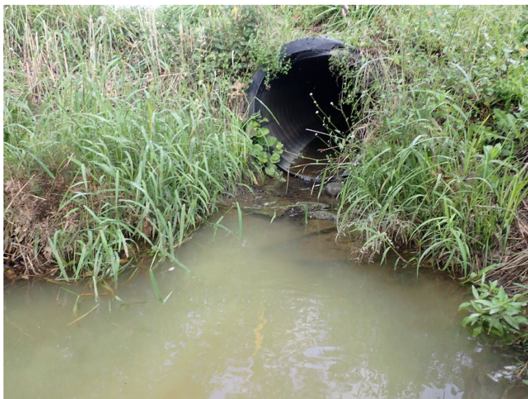
Photograph IV.D. Excavated Wetland 16 tributary culvert. Facing north.
