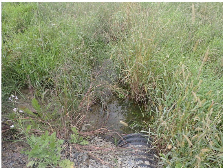
Photograph XIII.G. Second culvert draining Wetland 8. Facing South.
