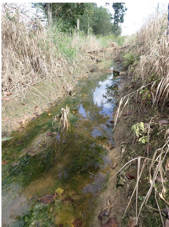
Photograph V.E. Excavated Wetland 16 tributary. Facing North.
