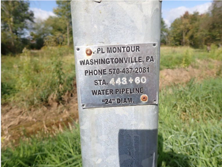
Photograph V.H. Water pipeline post, marking the boundary of the easement, at south end of excavated Wetland 16 tributary.
