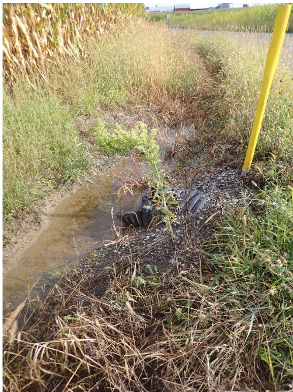
Photograph I.E. Culvert connecting flowing water between corn field and Mill Road to swale on northwest corner of Wetland 19. Facing North.
