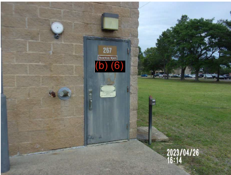
Photograph 56: Building 267 Central Accumulation Area (CAA)
