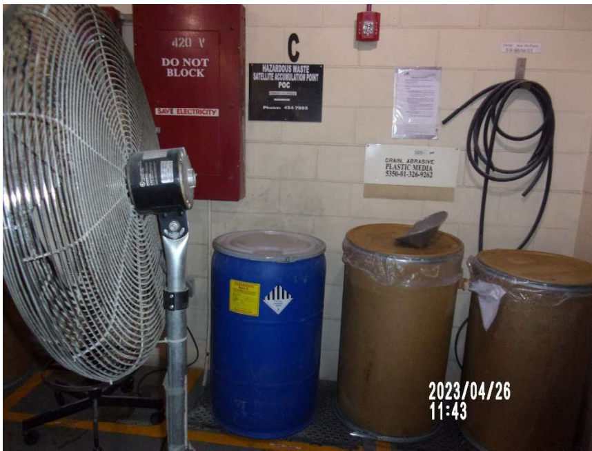
Photograph 11: Building 218 SAA C
