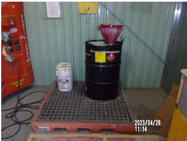
Photograph 1: Liquid Hazardous Waste in Building 220, SAA A
