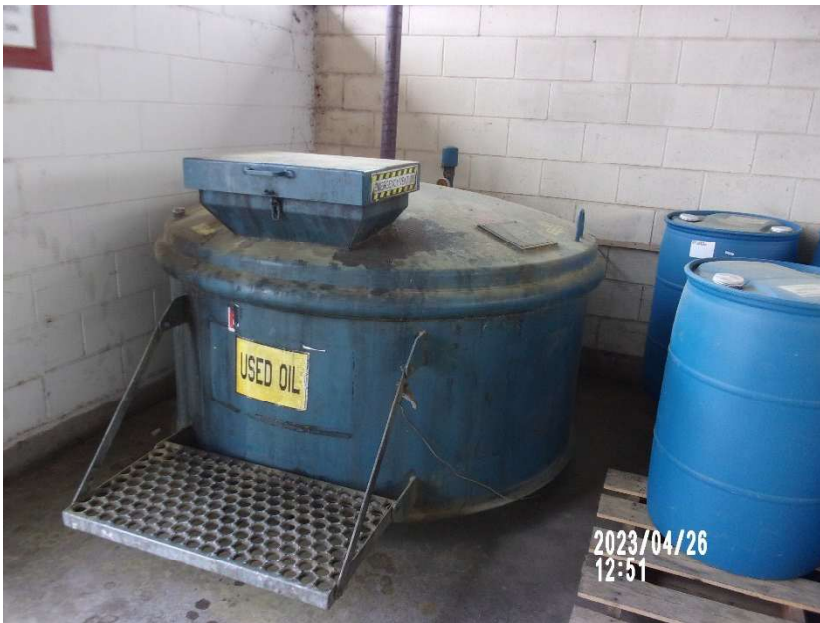
Photograph 30: Building 449, Used Oil Container
