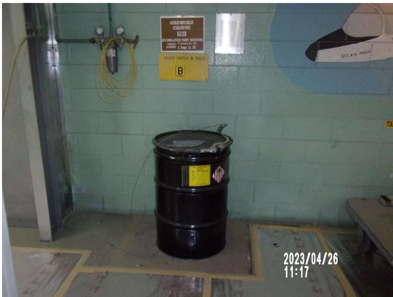
Photograph 3: 55-Gallon Container of Hazardous Waste Solids in Building 220, SAA B
