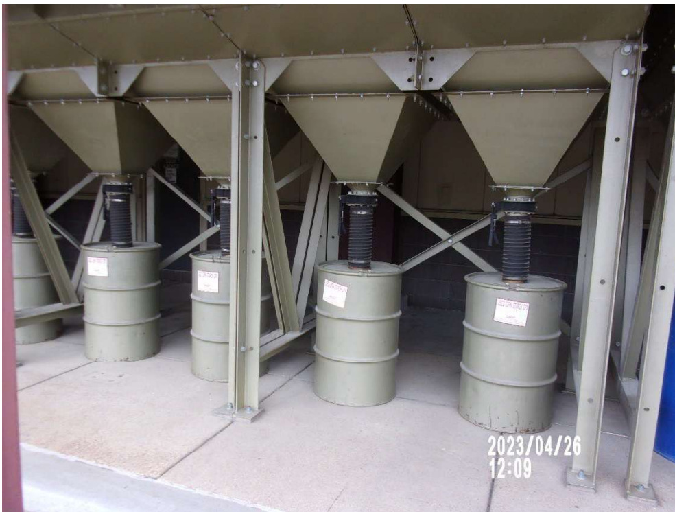
Photograph 18: Building 414 – Blast media collection
