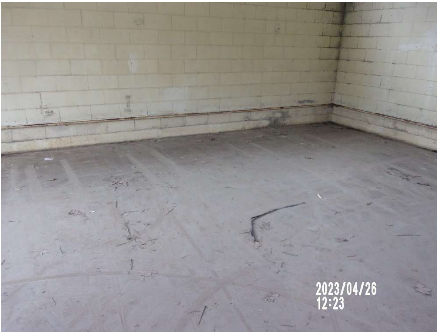
Photograph 23: Empty Space in Building 265 CAA
