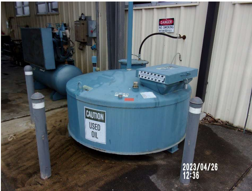
Photograph 26: Building 410 Used Oil Container
