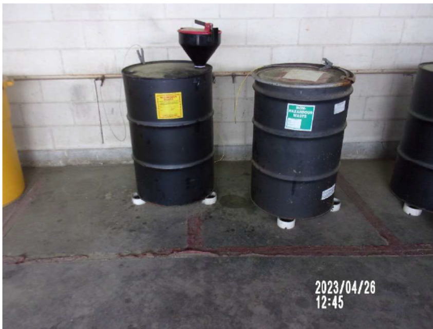
Photograph 28: Building 449, SAA A, Container Missing Hazard Indicator
