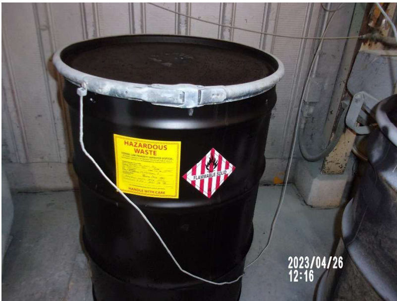
Photograph 20: Hazardous Waste Label and Hazard Indicator on Solids Container
