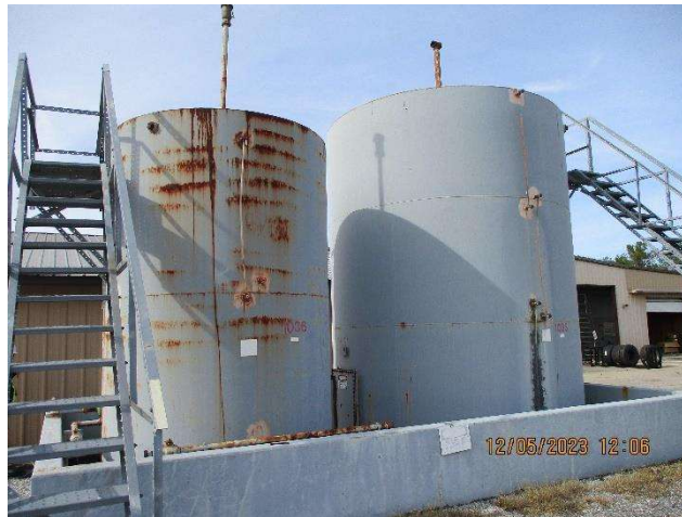
Photo # 6 General view Tanks 1035 and 1036
