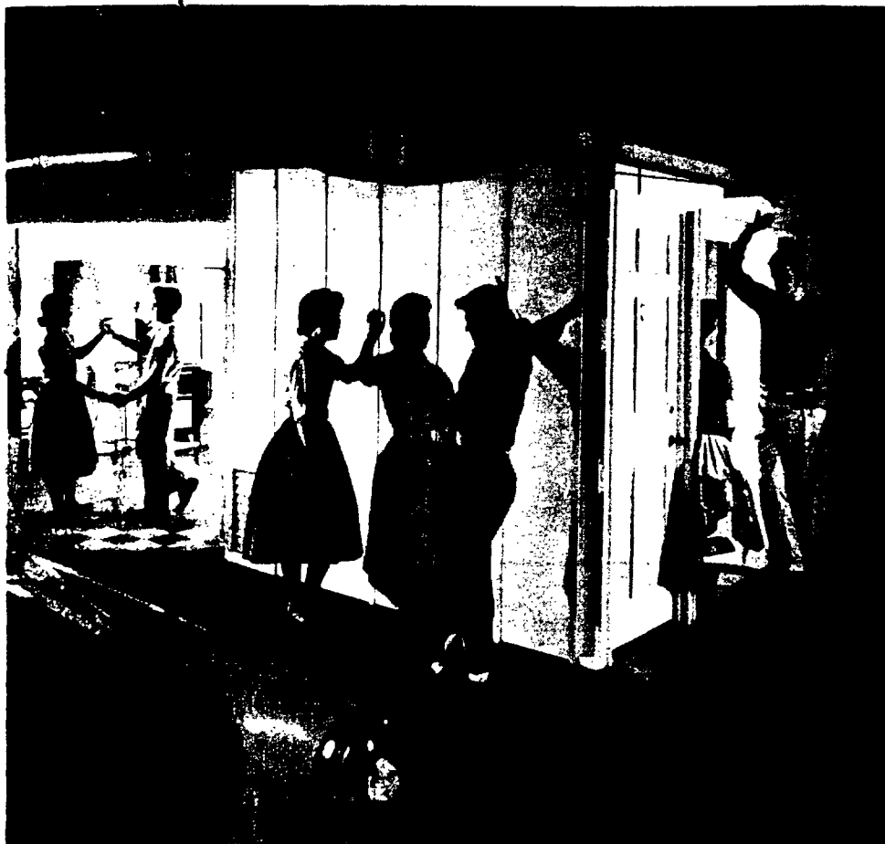
On the garage side of new partitions, studs were faced with boards and batten strips. Folding doors provide ventilation, and a place to lean. The single door opens to stairway.
