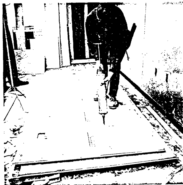
Applying Grabit to Dens-Cote Base
