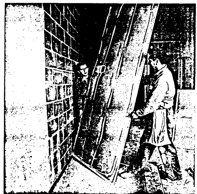
Installing Dens-Cote Base on Masonry Wall
