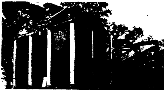
Destroyed by the hurricane, lead flashings and white lead paint will help to restore this stately church to its original beauty ←
