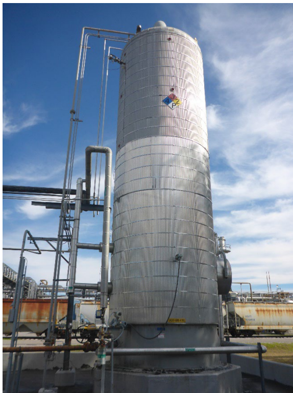
Photo 2: Hazardous Waste Storage Tank 007-08-415.
