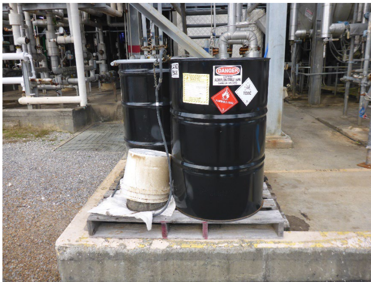
Photo 8: One 55-gallon drum, which was labeled hazardous waste (acrylonitrile, styrene) and identified as flammable and toxic, in the Line 4/5 Decanter SAA.
