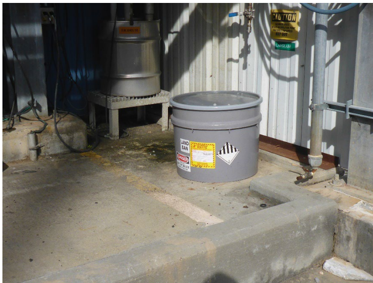
Photo 10: One 20-gallon container, which was labeled D001, F005 hazardous waste solid (MEK), in the second Pilot Plant SW End SAA.
