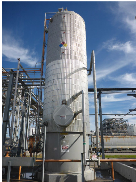
Photo 3: Hazardous Waste Storage Tank 007-25-027.
