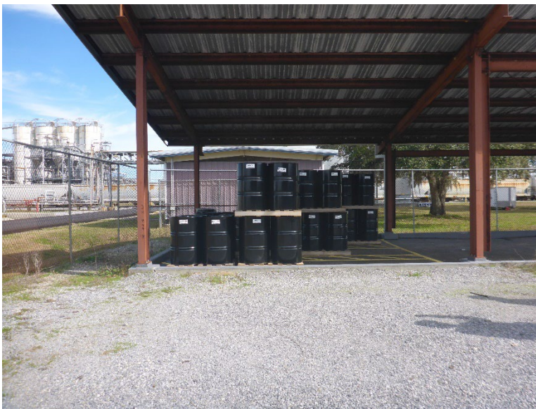
Photo 6: Nonhazardous waste storage area.
