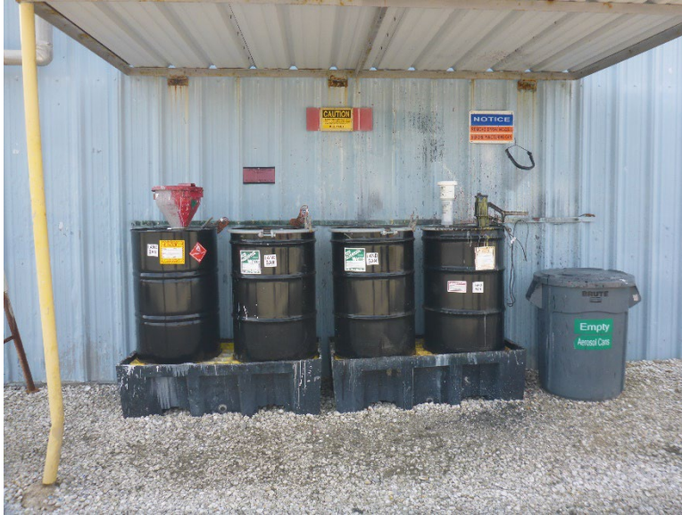
Photo 11: One 55-gallon drum, which was labeled D001, F005 hazardous waste used paint (MEK) and identified as flammable, in the first Maintenance Paint Shop SAA on the left pallet; and one 55-gallon drum, which was labeled D001, F005 hazardous waste flammable liquids (toluene, MEK) and identified as flammable, in the second Maintenance Paint Shop SAA on the right pallet.
