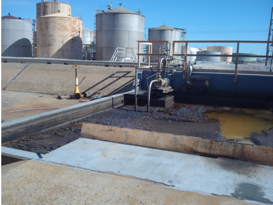
Photograph 3. Hazardous waste drying pad with solids from Sumps 21, 22, and 24 (truck and rail loading/unloading area).
