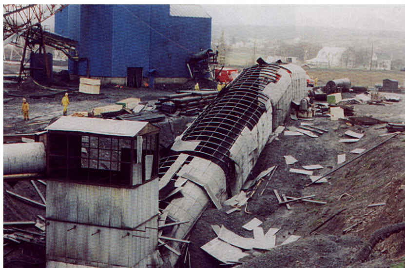
Figure 8. Damage to portal at No. 1 main, Westray coal mine. 29
