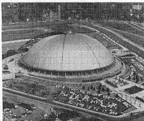
Roof closed, arena is cool in summer, snug in storms.
