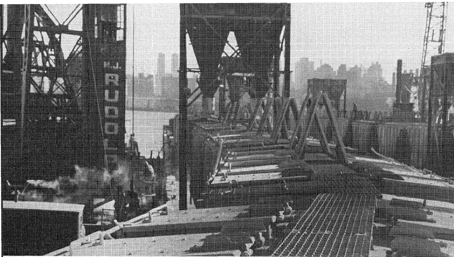
Corrosion is relentless enemy of covered hopper cars and their costly loadings. New Du Pont coating system will protect car and contents.
