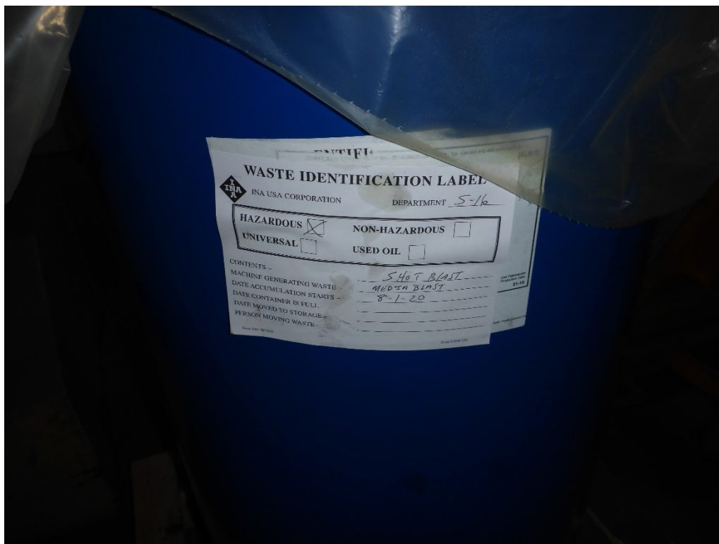
Photo 3: 55-gallon blue poly drum in the spent shot blast media SAA. The waste identification label identifies the material as hazardous shot blast media blast.
