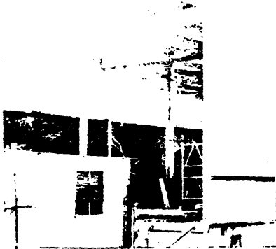
(Above) Kaylo Laminated Panels provide a neat outside wall, resistant to fire and weather.
