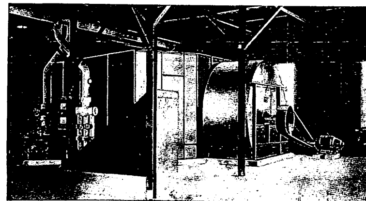
Typical Installation of Buffalo Fan and Carrier Air Conditioning Equipment
