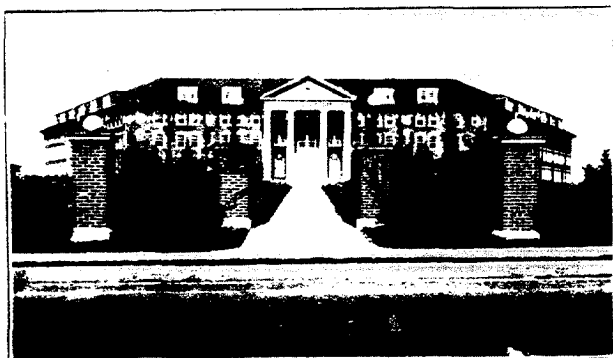
Glistening T.T.O. Outside White embellishes the pillars and window frames of Penn Hall School at Chambersburg, Pennsylvania. Liquid Velvet lends soft, durable beauty to the interior of this fine building.
