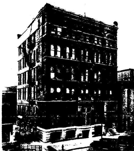
T.T.O. PAINT, Light Green was used to finish all window frames in the big Salvation Army office building in Omaha. These frames had not been painted for many years, but one coat did the job! Shrier Paint and Wallpaper Co. sold this job.
