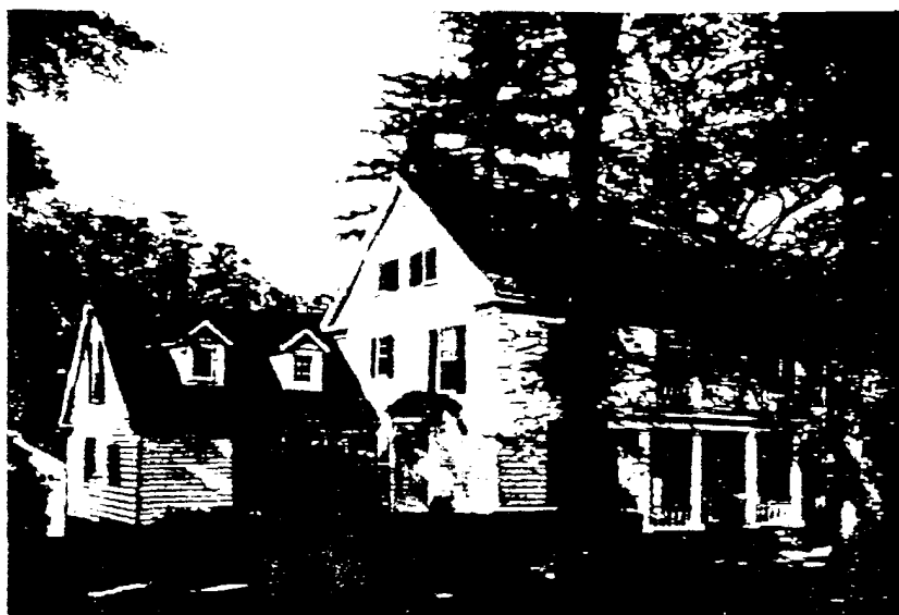
The Griffin House, the oldest house in Cooperstown shows the characteristic whiteness of self-cleaning pure white lead paint.
