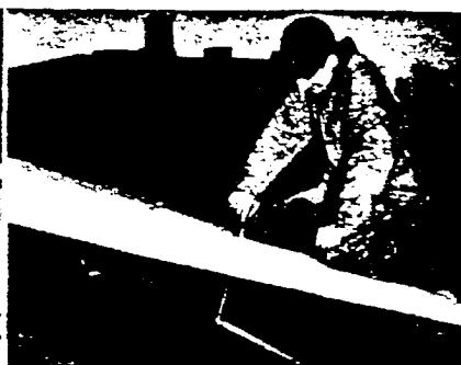
Left. The threaded steel rod is inserted into the hole in the asbestos roofing and hooked to the cross beam. Center. The lead seal and tab in place and the entire unit bolted together. Right. After folding the lead tab over the bolt it is hammered down.
