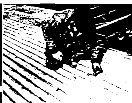
Left. The threaded steel rod is inserted into the hole in the asbestos roofing and hooked to the cross beam. Center. The lead seal and tab in place and the entire unit bolted together. Right. After folding the lead tab over the bolt it is hammered down.
