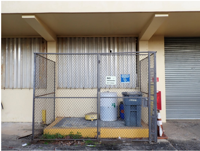
Picture 49 — Former Hazardous Waste Tanks Area—At the time of the CEI, ongoing construction activities were not observed since construction activities were completed by the day. It consists of a high galvalume ceiling with part concrete, and part soil floor. A yellow band that works as a physical barrier in order to control access to the latter was observed.
