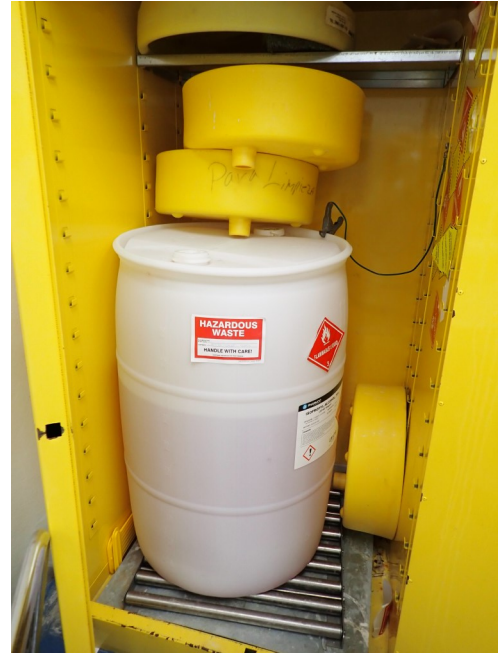
Picture 38 — Room M15 Washroom Area - Here, one (1) 55-gallon white plastic container with alcohol waste 70% was observed. It was closed, labeled as hazardous waste, has a pictographic label, and grounded.
