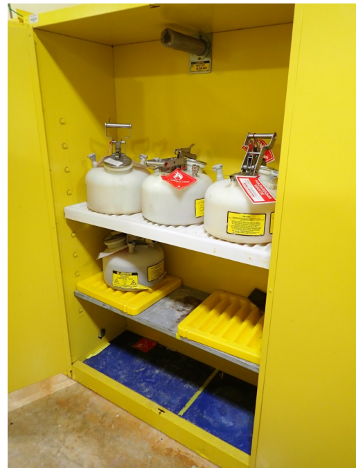
Picture 44 — Laboratory Area-Chemical Storage Q3 Area— Here, one (1) yellow shelf labeled as flammable and Full HPLC Safety Cans no halogenated waste was observed. Inside, the latter had four (4) 2.5-gallon white plastic containers.
