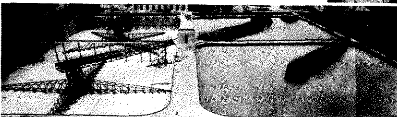
FIGURE 6 (lower right). FLOCCULATOR-CLARIFIER IN A SINGLE CYLINDRICAL TANK
