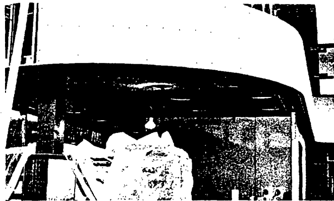
UNDERCOVER WORK —island takes shape as first layer of \frac{1}{4} -in. SHEETROCK wallboard rounds out framework. Face paper was dampened until wallboard would bend to curve. Second layer is laminated with PERF-A-TAPE joint compound.
