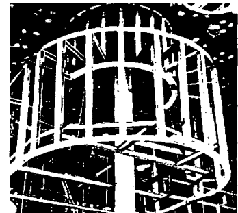
UNDERCOVER WORK —island takes shape as first layer of \frac{1}{4} -in. SHEETROCK wallboard rounds out framework. Face paper was dampened until wallboard would bend to curve. Second layer is laminated with PERF-A-TAPE joint compound.
