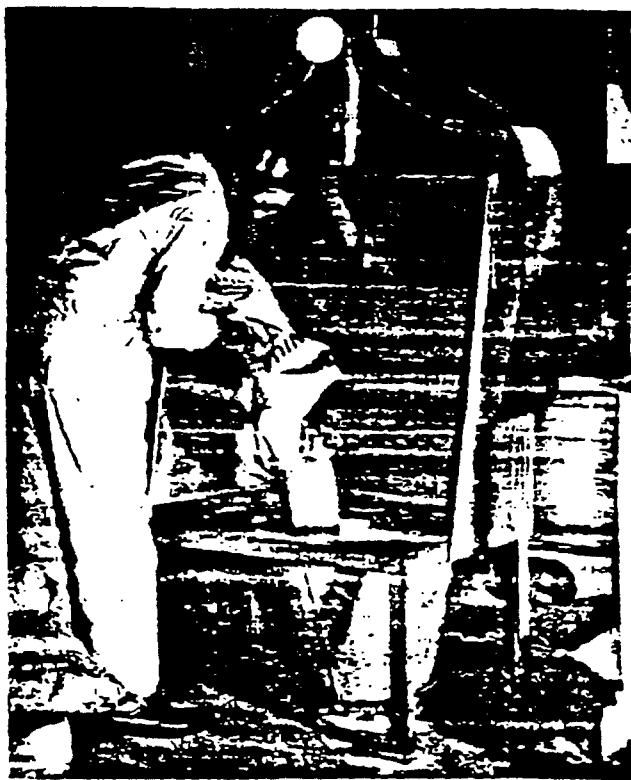
It should be a part of any occupational health program to educate employees in the correct handling of materials and to warn of the hazards of excessive exposure. Here, a kettle is being charged with a chemical which generates toxic dust. Note use of respirator, gloves, ventilating equipment, and coverall.
