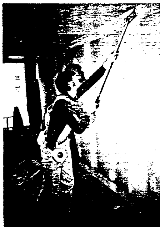
Figure 1 — Pole sanding of drywall taping compounds. Several applications of taping compounds may be required to make a smooth joint between gypsum wall boards, requiring extensive sanding.
