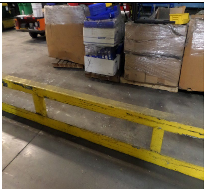
Facility Maintenance Shop. The inspectors returned to this area and observed the two lead-acid batteries were managed for off-site disposal. Photograph 20 taken at 4:52 p.m.
