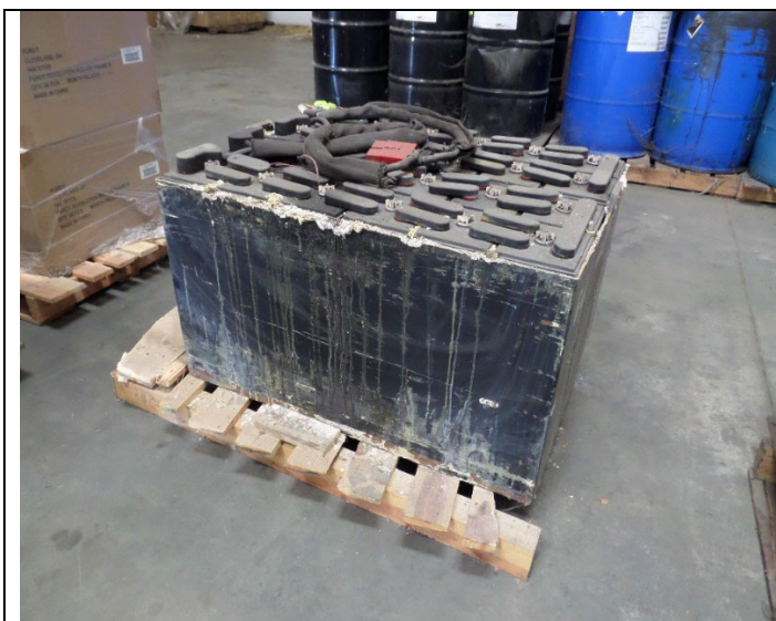
CAA. The inspectors observed one “sitdown equipment” battery leaking and not marked as universal waste and not dated. Facility managed the battery and shipped it off-site for disposal. Photograph 13 taken at 12:21 p.m.
