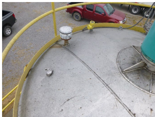
Photograph 34: Hazardous Waste Tank CAA.
