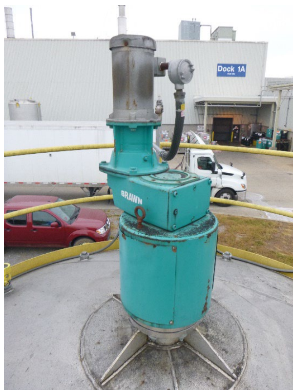
Photograph 35: Hazardous Waste Tank CAA.
