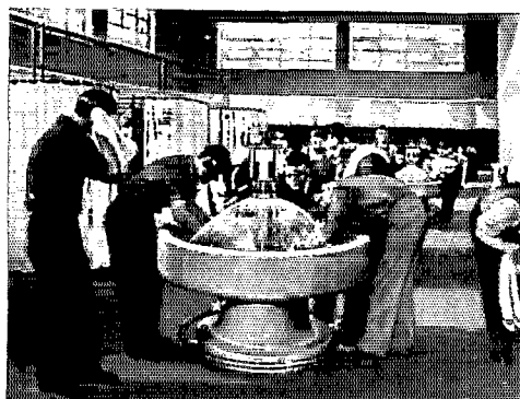
Bradley Washfountains and, at left, three Bradley 5-Unit Showers.
