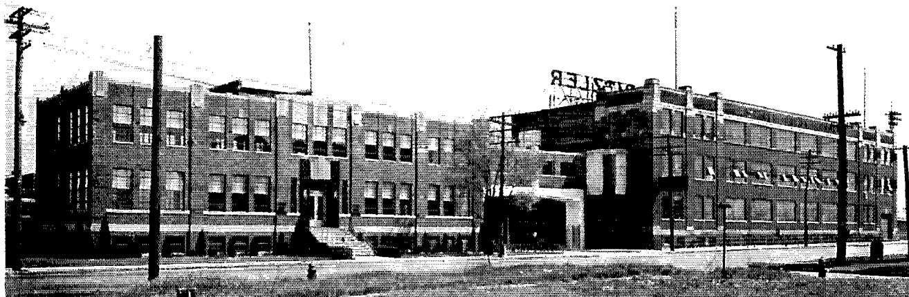
The neat, trim exterior of the plant reflects what the visitor may expect inside.
