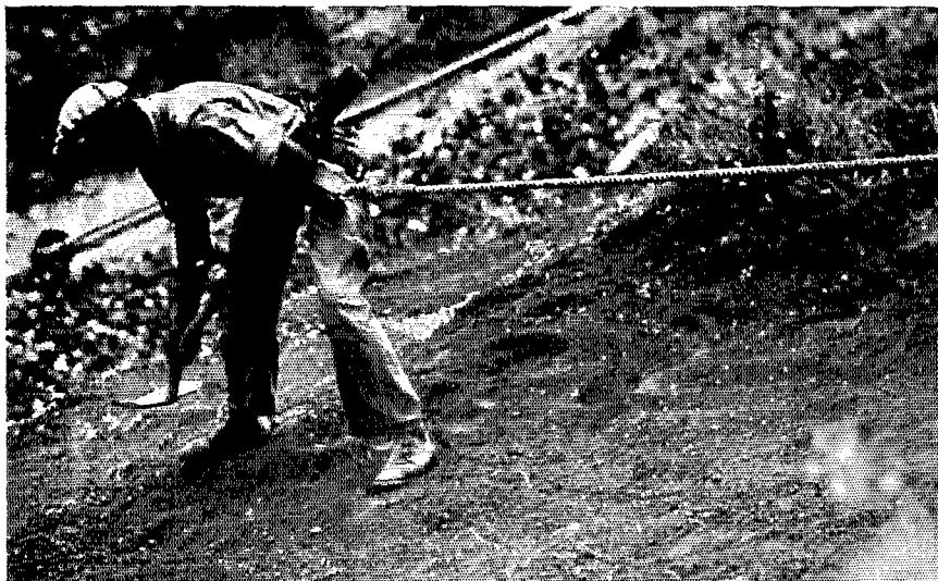
Courtesy Tennessee Valley Authority This man is working within six inches of the brink of a 60 foot cliff. The safety belt and life line will save him if the earth gives way.
