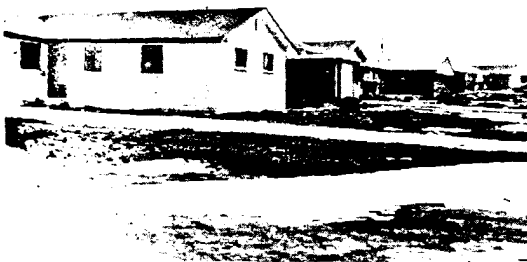
The homes of the Carey Carnation Development in Aurora, Colo., are medium priced single-family ranch homes. Lead fixture connections and waste lines were installed as they were in . . .
