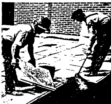
Weatherwood Roof Insulation
