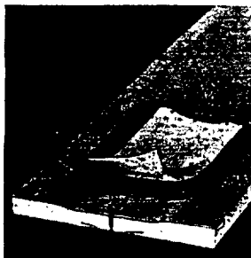
Perfatape Joint Treatment over Recessed-Edge Sheetrock
