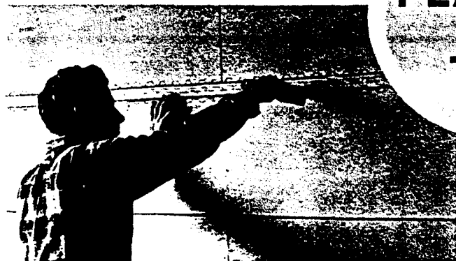
Keystrip adds extra strength to points of stress
