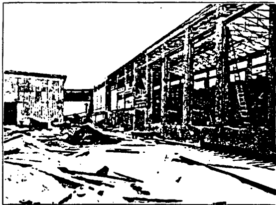
Structolite Curtain Walls on Portland Cement Foundation
