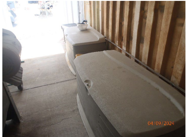
Picture 32 – Universal Waste Batteries
