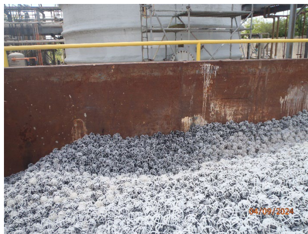
Picture 25 – TOU Roll-off packing from air strippers
