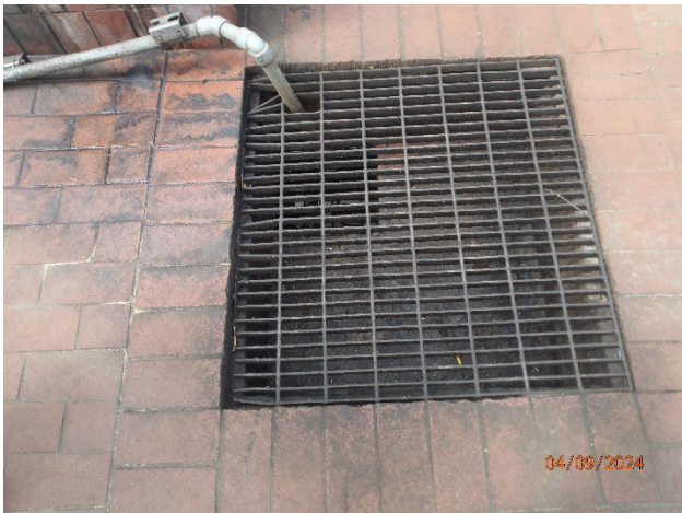
Picture 13 – HW tote unloading sump
