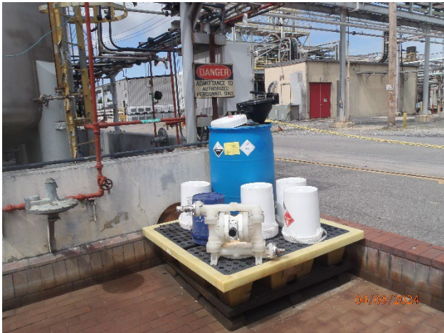
Picture 12 – HW tote unloading area
