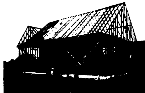
Five rooms, 27' 0" x 36' 0" ready for Gyplap
