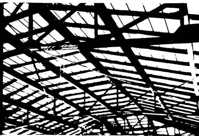
Underside of Sheetrock Pyrofil roof, illustrating the high light reflection quality of this construction.
