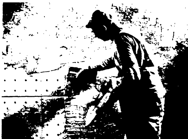
Perforated Rocklath provides an additional bond for plaster with its regularly spaced perforations.
