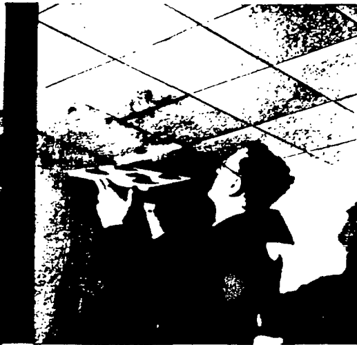
Weatherwood Tile applied with adhesives to flat surfaces.
