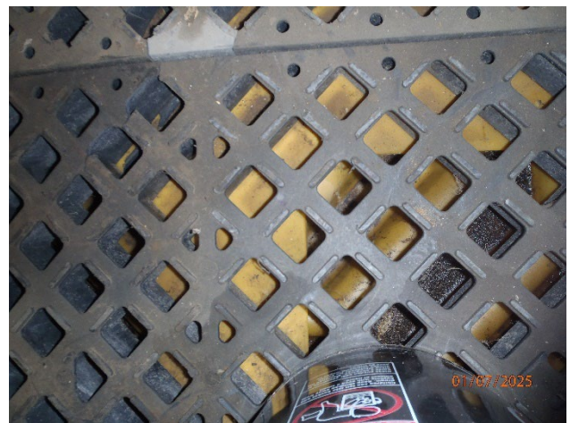
Picture 23 – Maintenance oil center containment pallet
