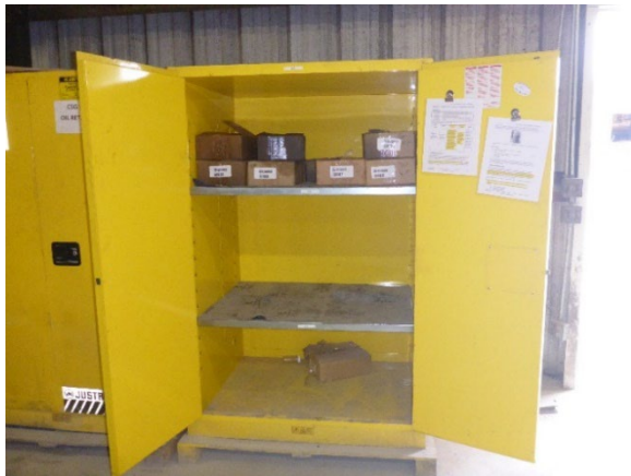
Photo 9 (Product Storage Warehouse SAA): Flammable locker containing boxes of used oil sample retains and hazardous waste used oil sample retains.
