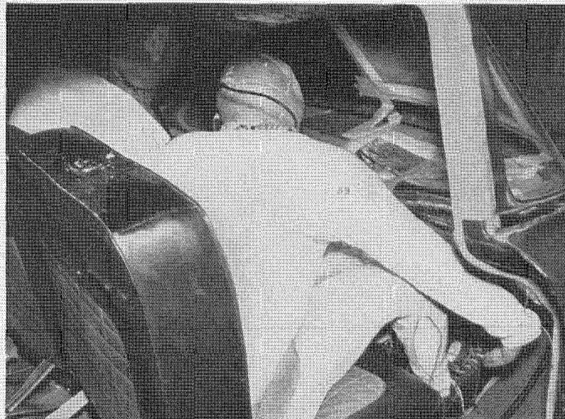
Ford Motor Co. staged automobile crash-ups using life-size dummies to test the effectiveness of such safety devices as protective padding.
