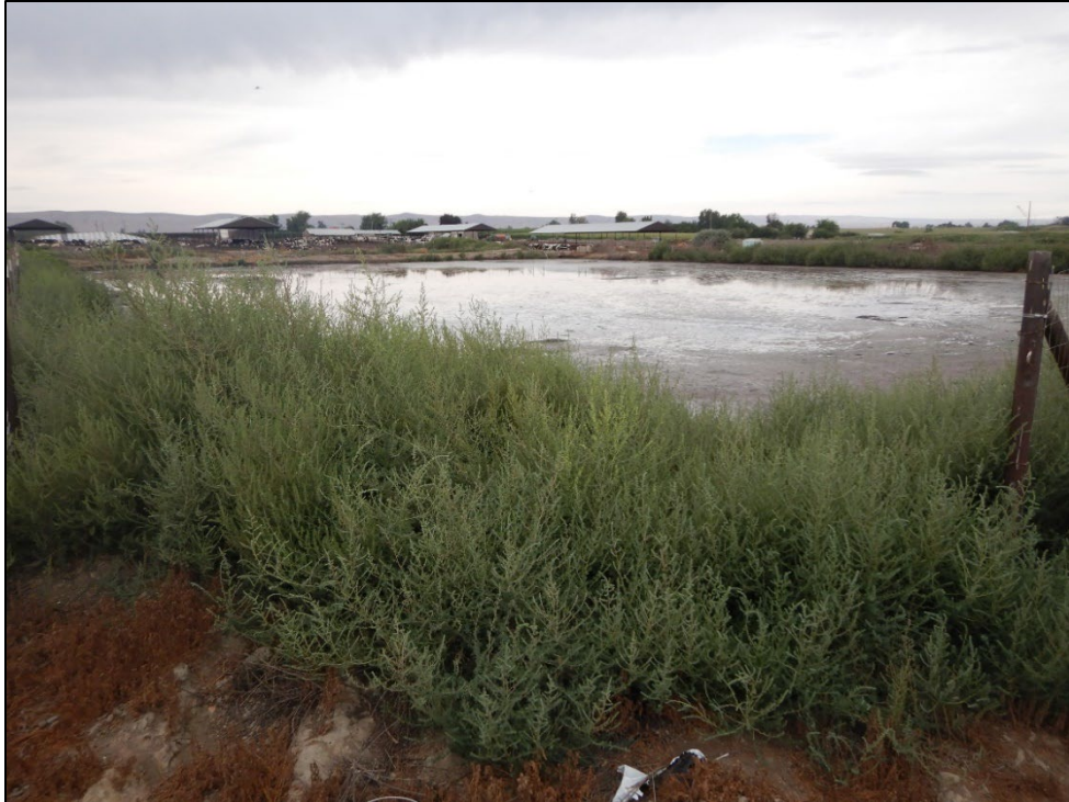
Photograph 15. View looking southwest across Lagoon 2. Note the heavy vegetation growing on the embankments.
