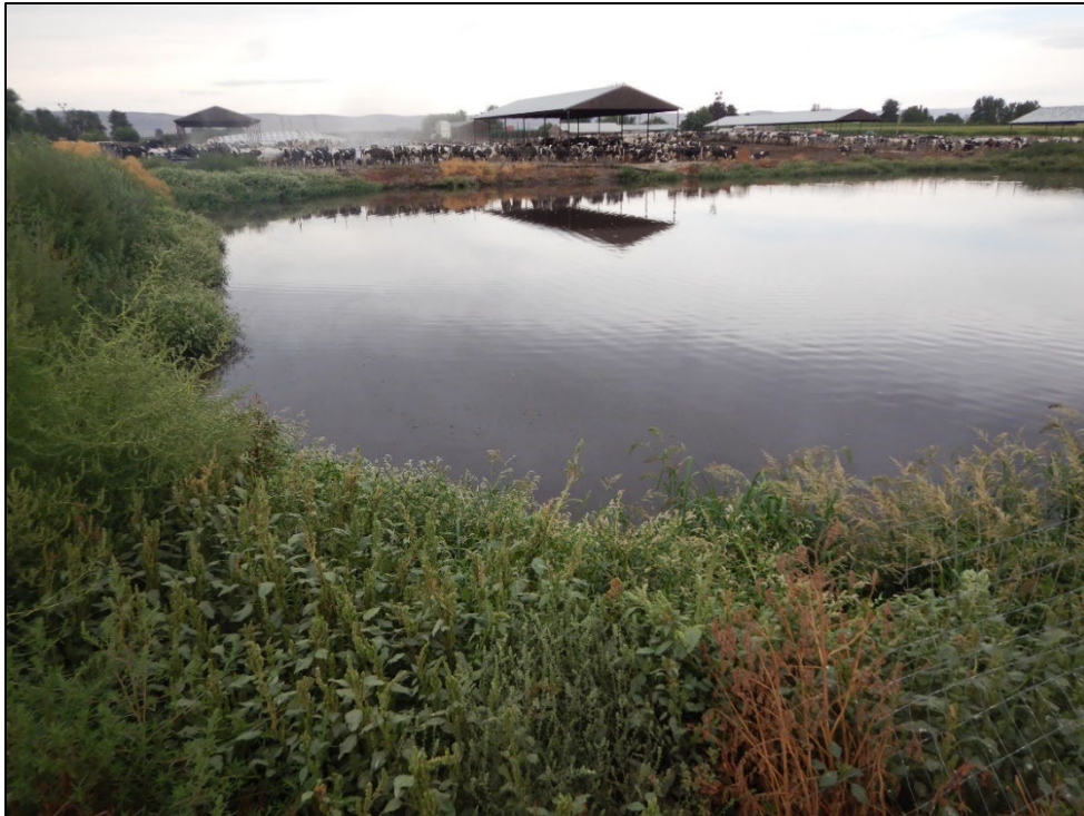
Photograph 19. View looking southwest across Lagoon 1. Note the heavy vegetation growing on the embankments.
