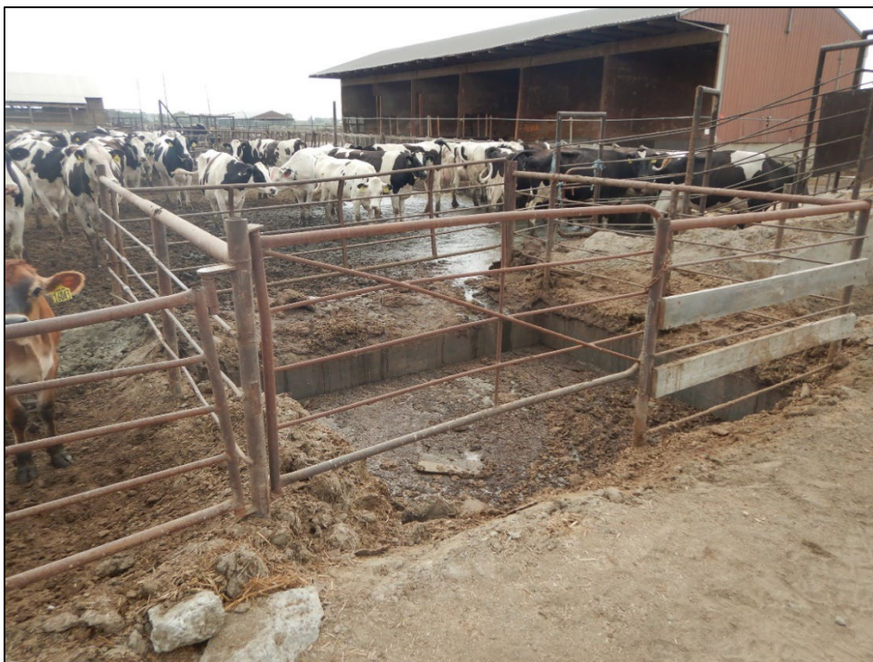
Photograph 2. View looking northeast at the concrete-lined West Silage Pit.
