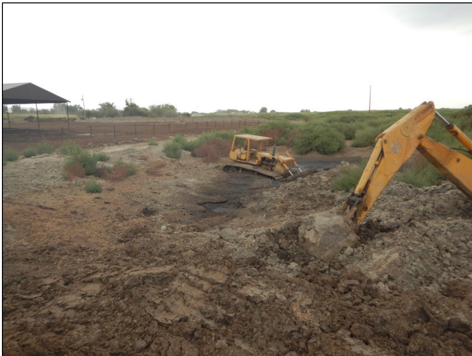
Photograph 28. View looking southwest at the low spot located west of the Settling Pit.
