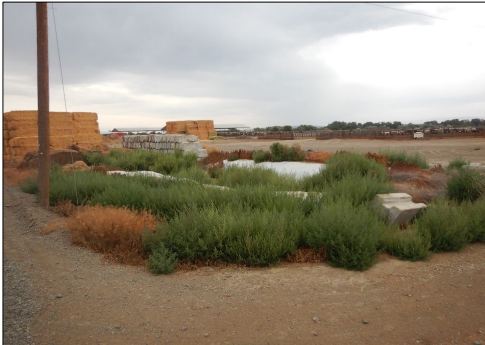
Photograph 6. View looking northwest of the East Silage Pit located at the southeast corner of the production area. The East Silage Pit was lined with a plastic liner, however, the inspection team heavy vegetation growing within the pit.
