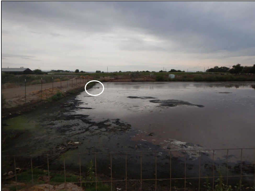
Photograph 17. View looking west across the southern portion of Lagoon 2. The PVC pipe (circled) is the overflow pipe between Lagoon 1 and Lagoon 2.
