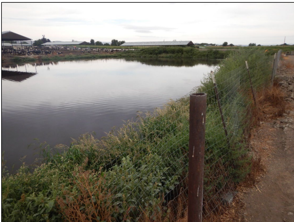
Photograph 20. View looking west along the northern edge of Lagoon 1. Note the heavy vegetation growing on the embankments.
