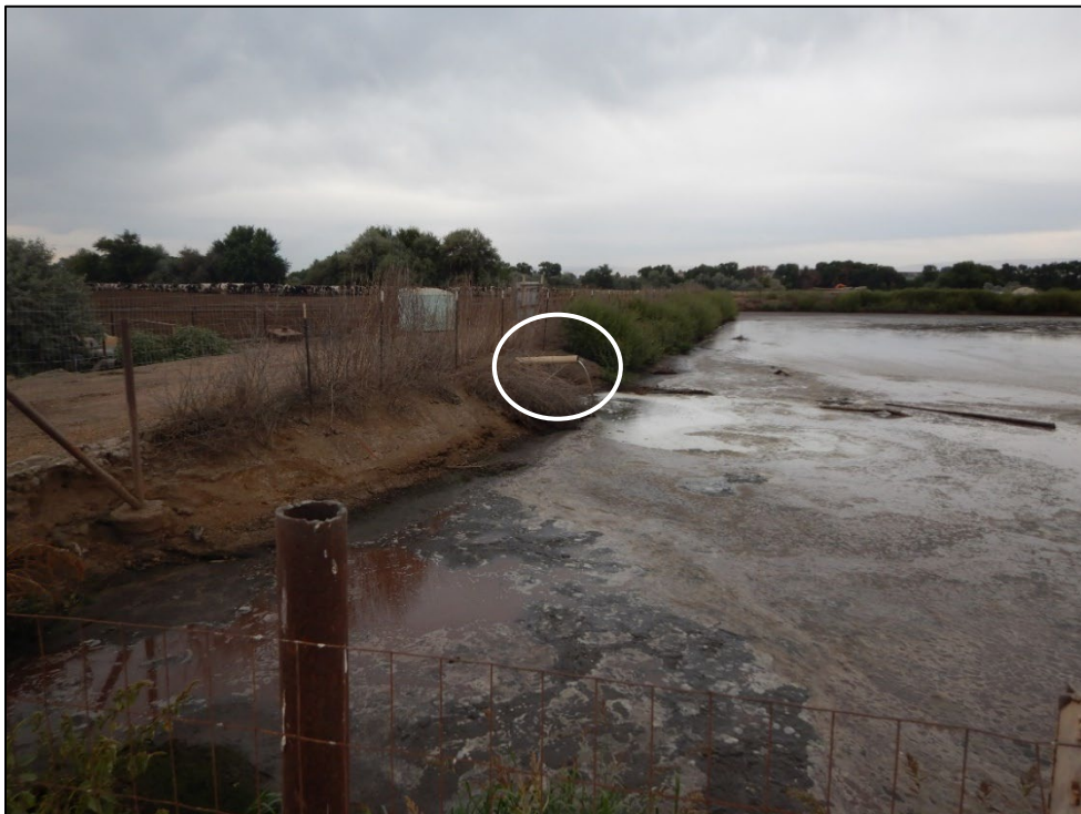
Photograph 26. View looking north at the PVC pipe (circled), also shown in Photograph 18 , that conveys wastewater from the Settling Pit to Lagoon 2.
