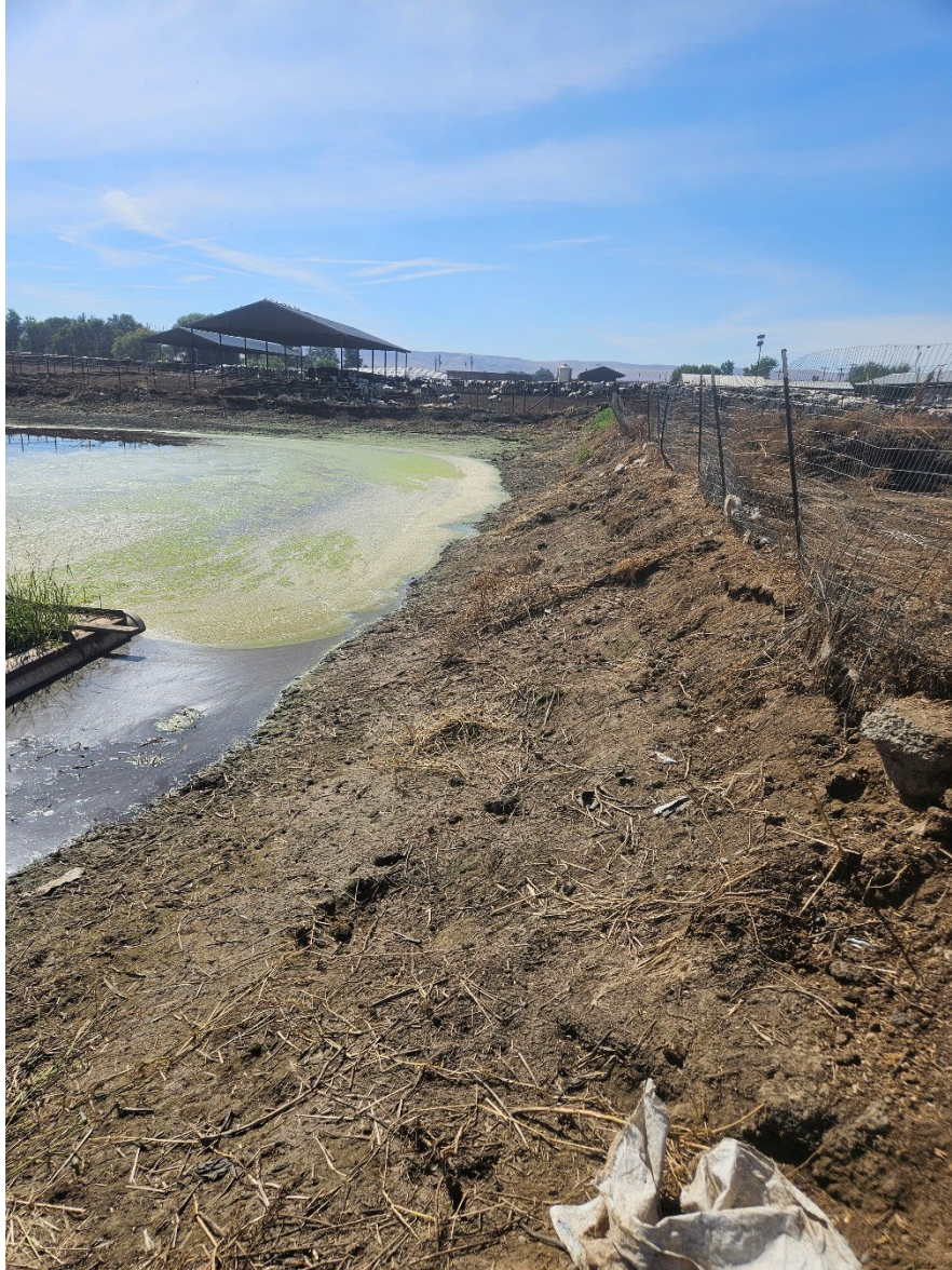
Photograph 3. View of Lagoon 1. Note the absence of vegetation compared to the photographs taken during the inspection site tour.
