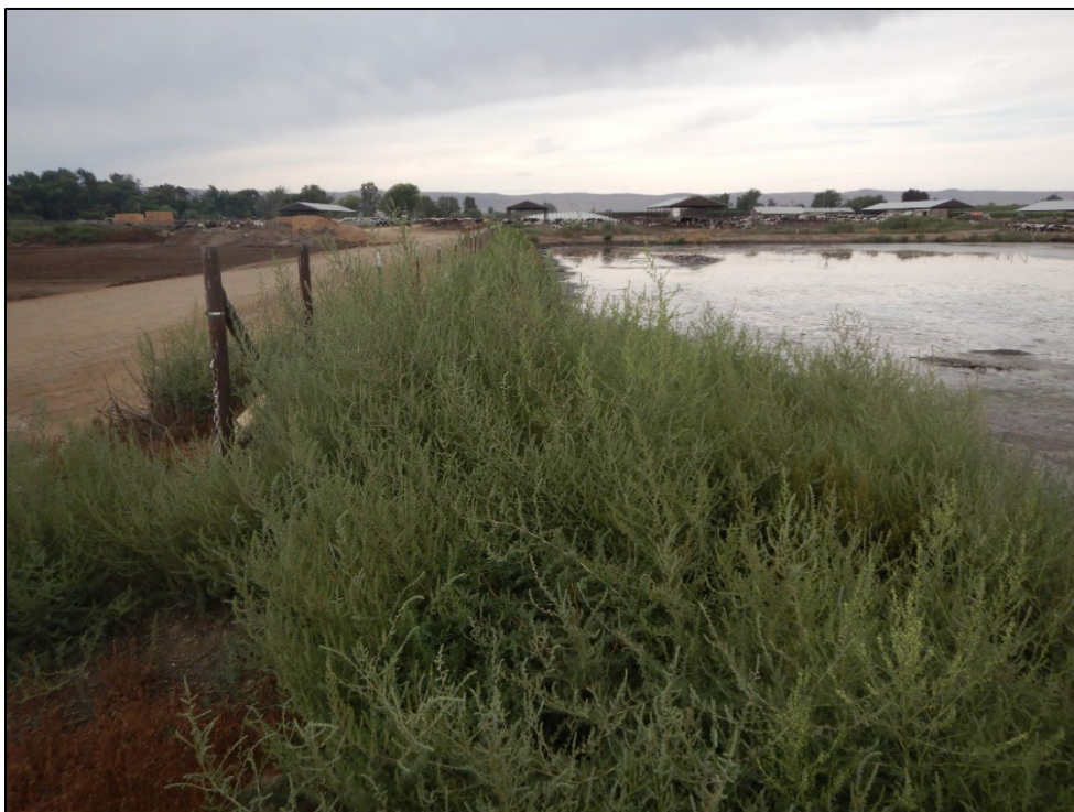
Photograph 16. View looking south, along the eastern edge of Lagoon 2.
