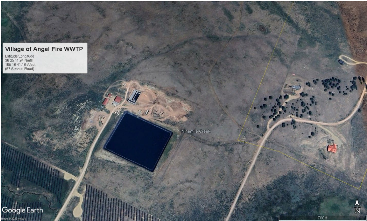
Aerial Image #1: Overall view of the Village of Angel Fire’s Wastewater Treatment Plant. Aerial from Google Earth maps.
