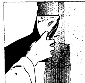
Forcing cement through perforations and leveling surface.
