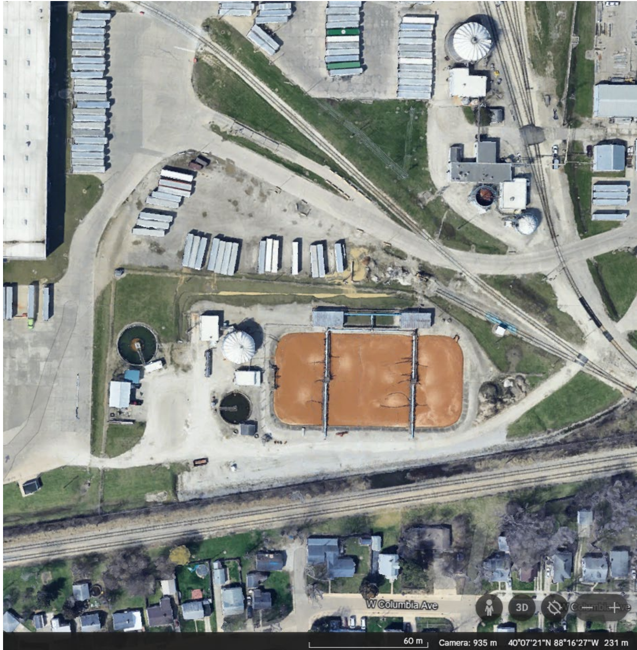
Aerial Image 1: Shows the wastewater pretreatment system at Kraft Heinz.
