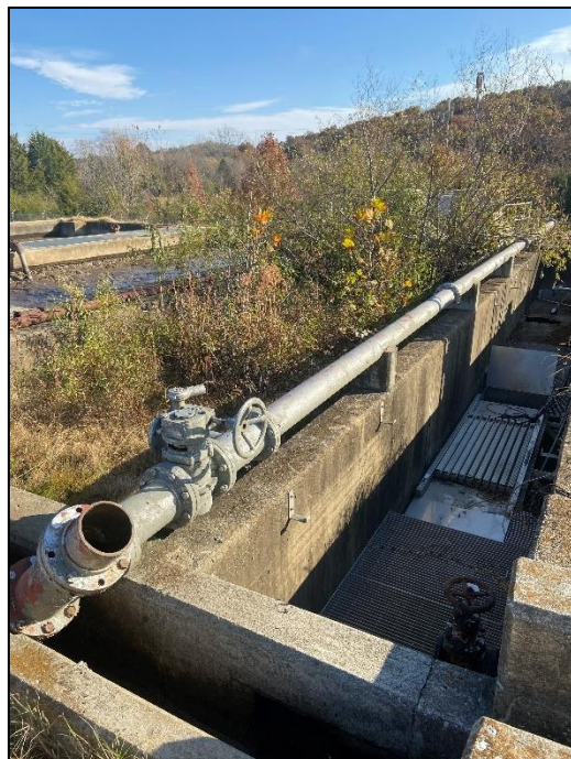
Photo 2: Return Activated Sludge line.
