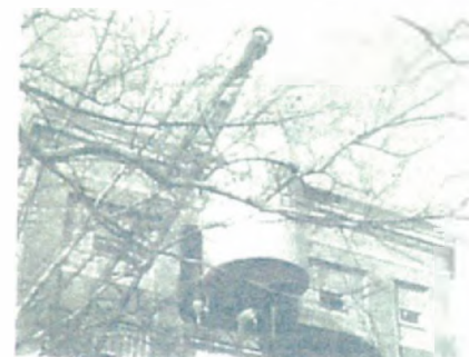
December 18, 1952 - first concrete mixer. Three mixers 1120 gallon processing tank, were taken from the fourth floor of the plant by means of a huge crane, then down to existing level, then, for placement in Morristown.
