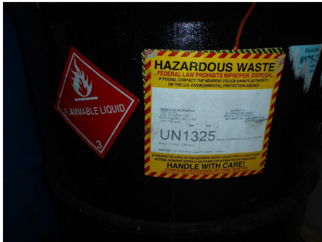
Photo 2 (P1010540.JPG): Hazardous waste container label Row 8 Flammable Storage Area.
