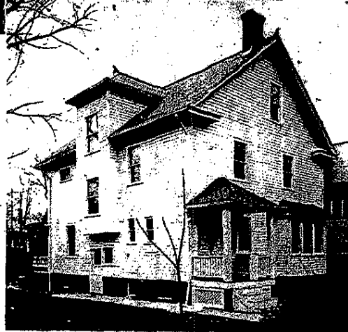
Top picture: Surface consisted of (1) 15-year weathered paint, (2) new siding patches (3) burn-off areas (spot primed).
