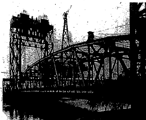
Bridge finished: One coat S-W Kem-Kromik Metal Primer, two coats S-W Kem-Elastic Metal Protective Paint.
