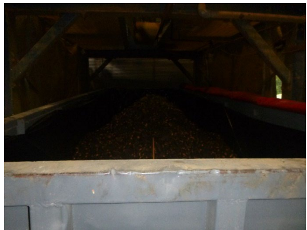
Photograph 58: Rimfire WWTP CAA 1-03.
