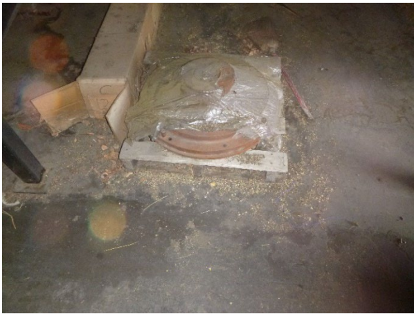
Photograph 73: Waste on floor near CAA 1-07.
