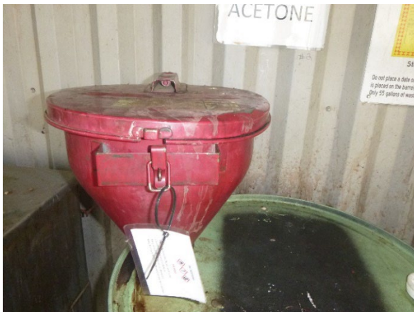
Photograph 56: Acetone SAA outside Loading.
