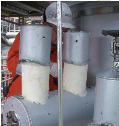
Picture 4 and 5: Cured foam after LP SPF injection.
