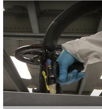
Picture 2: LP SPF pipe insulation
