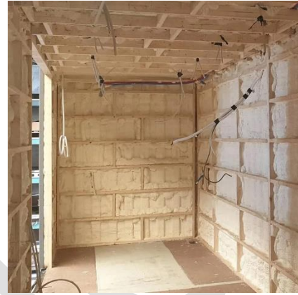
Picture 7: Container walls and ceiling insulated with LP SPF.
