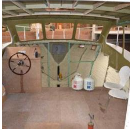
Picture 6: Boat wall insulated with LP SPF.
