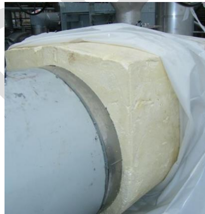
Picture 4 and 5: Cured foam after LP SPF injection.
