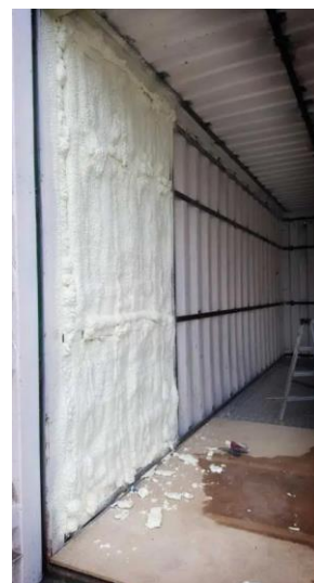
Picture 8 and 9: LP SPF application in limited space refrigerated transport containers.
