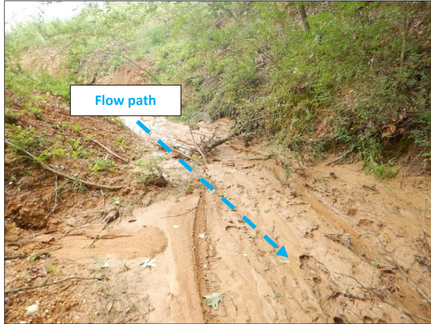
Photograph 59. Upgradient view of the stormwater flow path leading towards an unidentified discharge point in the center of the Site shown in Photograph 58 .
