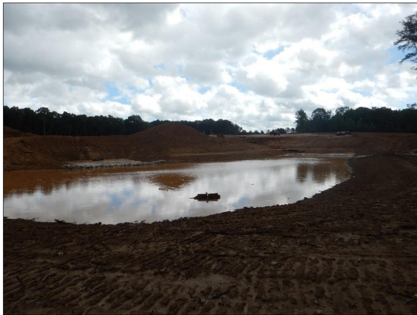
Photograph 18. View, facing east, of the sediment basin shown in Photographs 6, 7, 9, 10, and 15 . The basin contained sediment-laden water but no discharge occurring at the time of the inspection.
