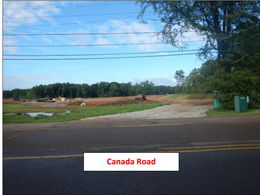
Photograph 3. View, facing west, of the stabilized construction entrance/exit off Canada Road.
