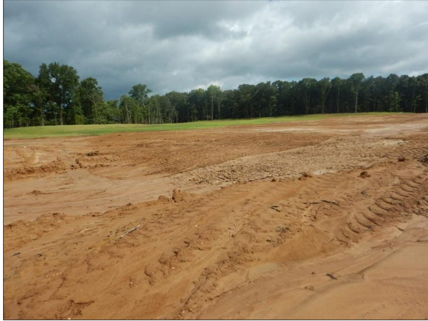
Photograph 5. View, facing west, of the northwestern portion of the Site. This area was actively under construction at the time of the inspection.
