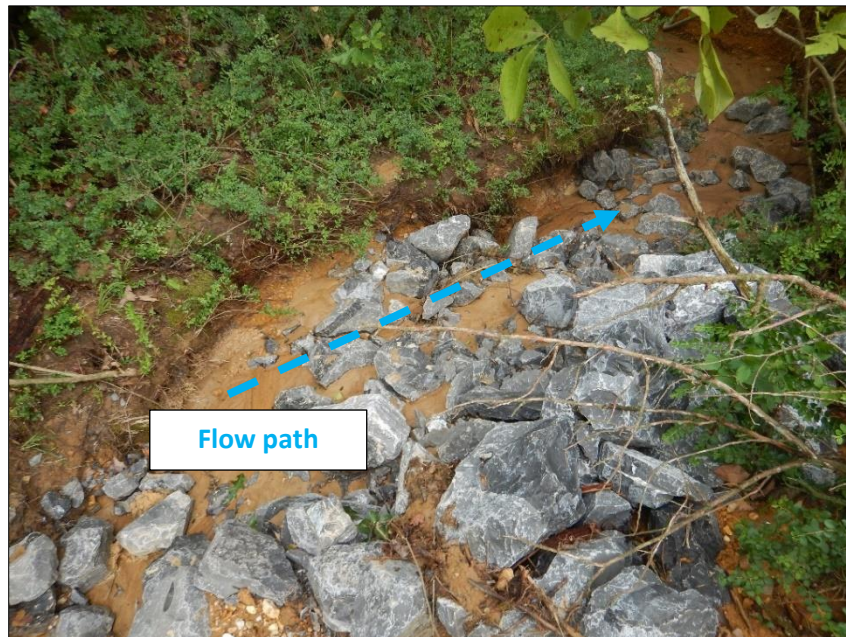
Photograph 60. View of offsite sediment discharge towards the unnamed tributary to Oliver Creek in the center of the Site.
