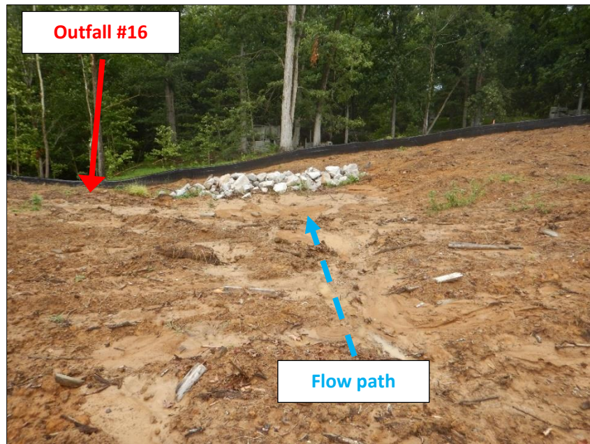
Photograph 38. Downgradient view of the flow path towards Outfall #16 in the center of the Site. Silt fence was installed across the channel downgradient from Outfall #16, an area of concentrated flow.
