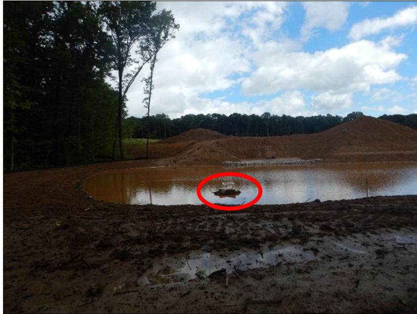
Photograph 15. View, facing east, of the sediment basin shown in Photographs 6, 7, 9, and 10 . The riser (circled in red) in the middle of the basin discharges through Outfall #5. The basin contained sediment-laden water but no discharge occurring at the time of the inspection.
