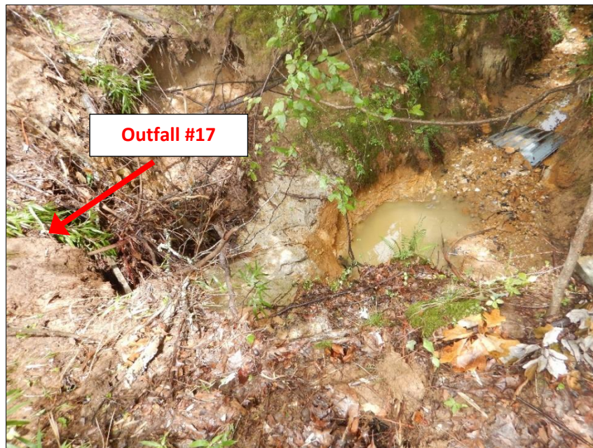
Photograph 36. Closer view of Outfall #17 and the head cut. The water leading to an unnamed tributary of Oliver Creek downgradient of the outfall was turbid.
