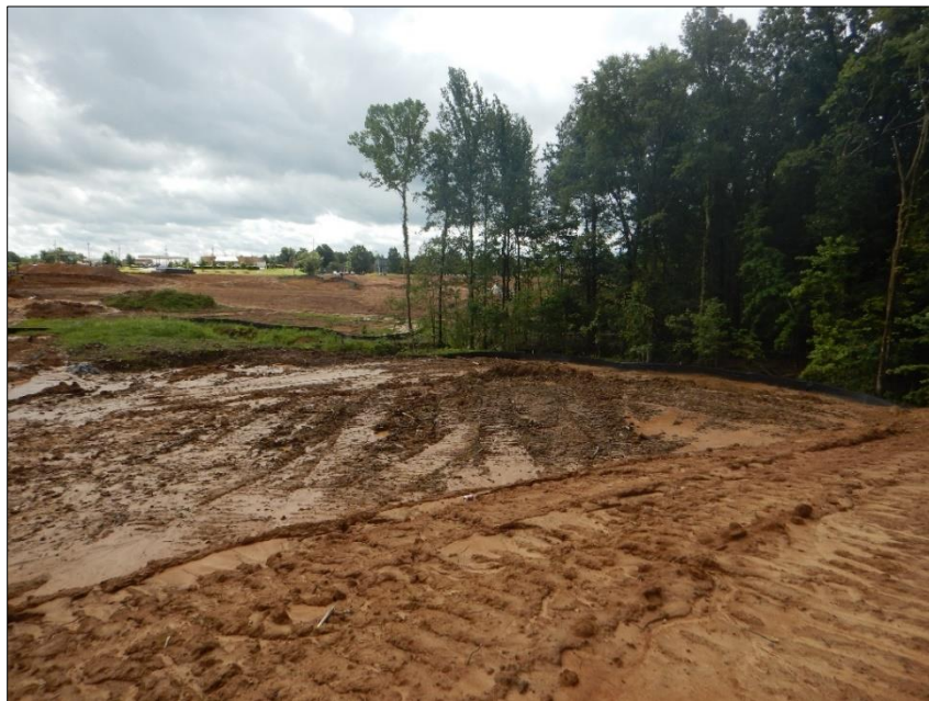
Photograph 22. View, facing south, of an active construction area in the western portion of the Site.
