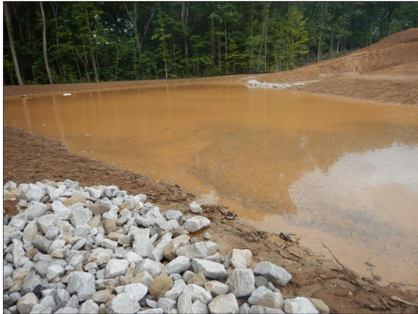
Photograph 10. View, facing northwest, of the sediment basin shown in Photographs 6, 7, and 9 . The basin contained sediment-laden water but no discharge occurring at the time of the inspection.
