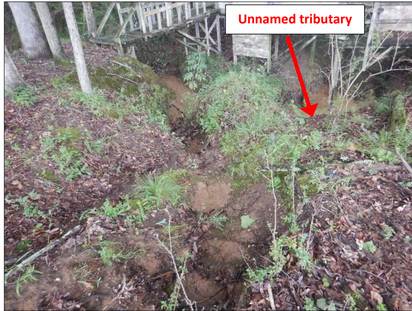
Photograph 45. Downgradient view of the erosion shown in Photograph 44 . The unnamed tributary to Oliver Creek runs adjacent to the Site in this location.
