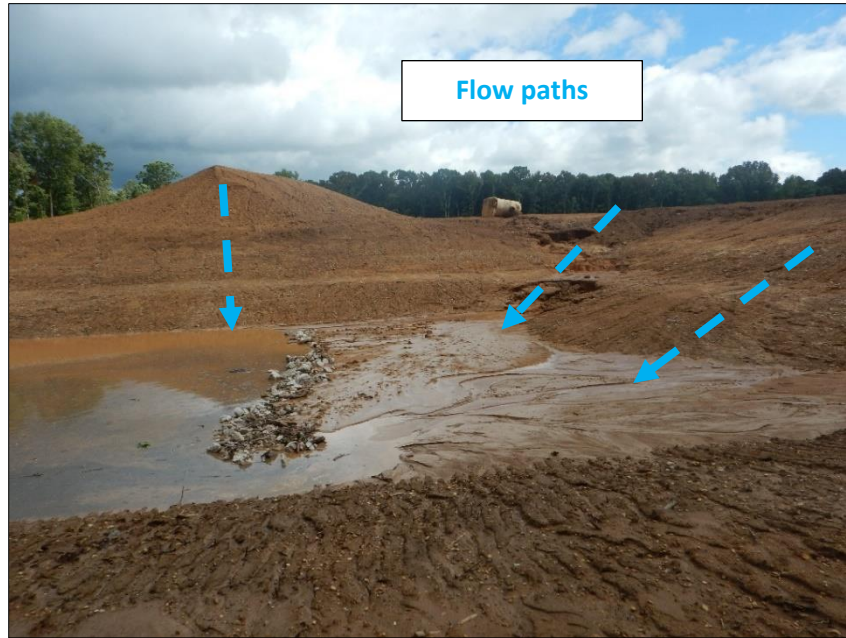
Photograph 9. View, facing north, of the basin shown in Photographs 6 and 7 . Rill erosion was visible on the unstabilized slopes leading to the basin.
