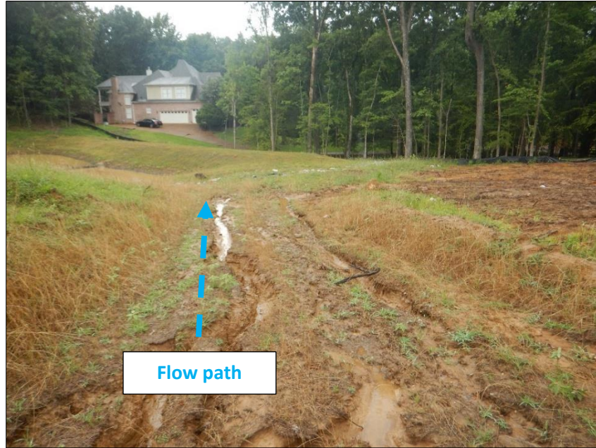
Photograph 33. Downgradient view of the stormwater flow path leading towards Outfall #18. Vegetative stabilization was not sufficient to prevent rill erosion on the slope leading to Outfall #18.
