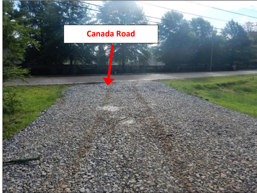
Photograph 1. View, facing east, of the stabilized construction entrance/exit off Canada Road.
