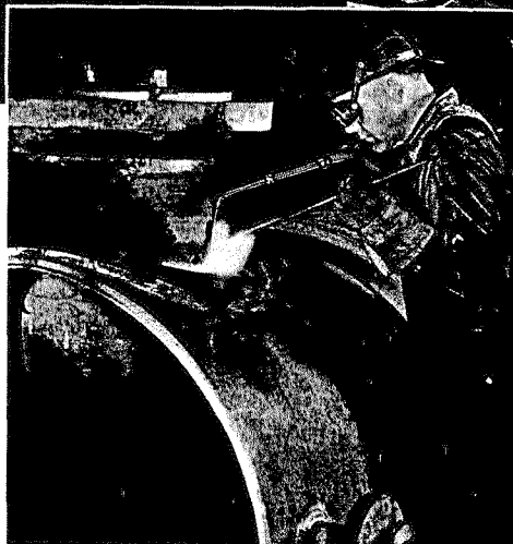
A welding operation on a special assembly in one of the fabricating shops.
